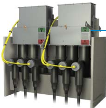
Floor Mounted Vault Installation
