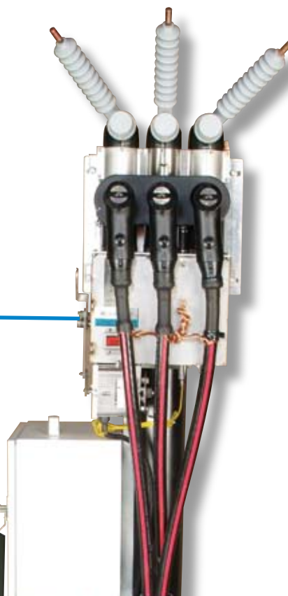
Riser Pole Installation
